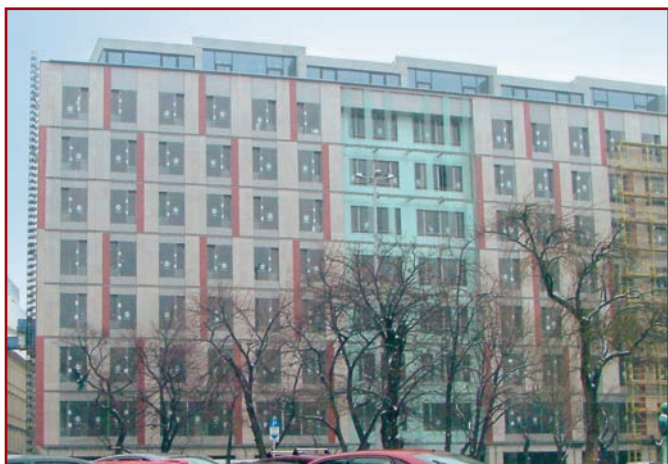
Roosevelt Office Building
