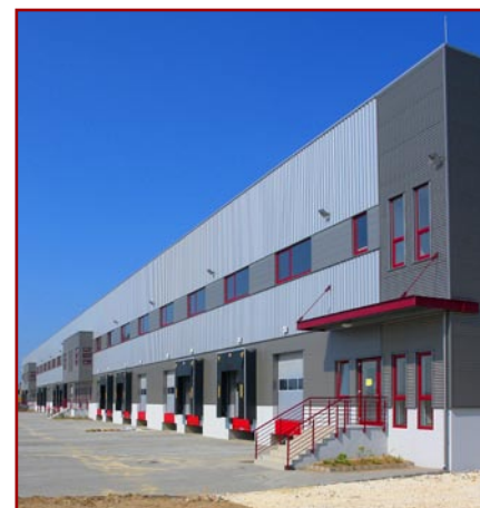
East Gate Business Park
