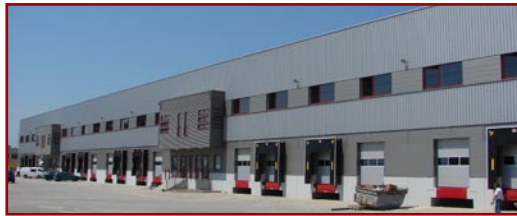
East Gate Business Park
