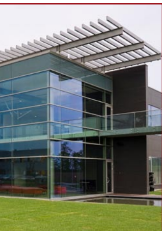
East Gate Business Park
